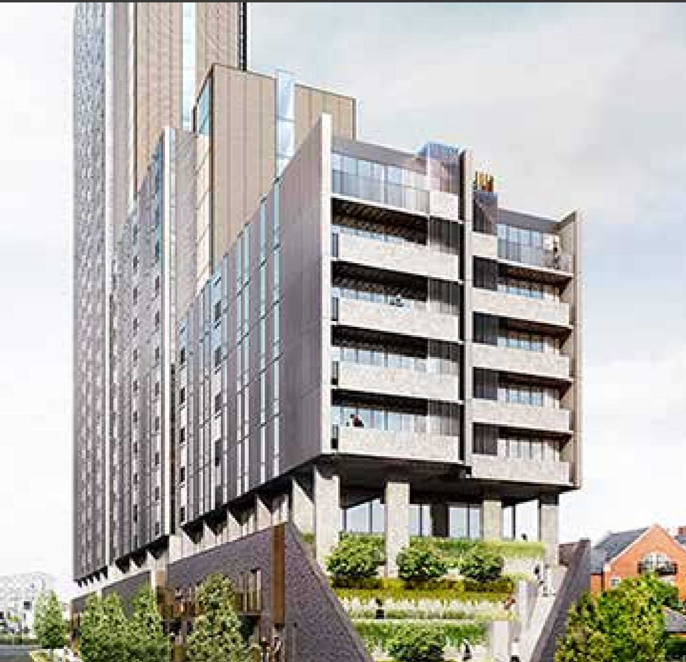
Oxygen Towers, Manchester
