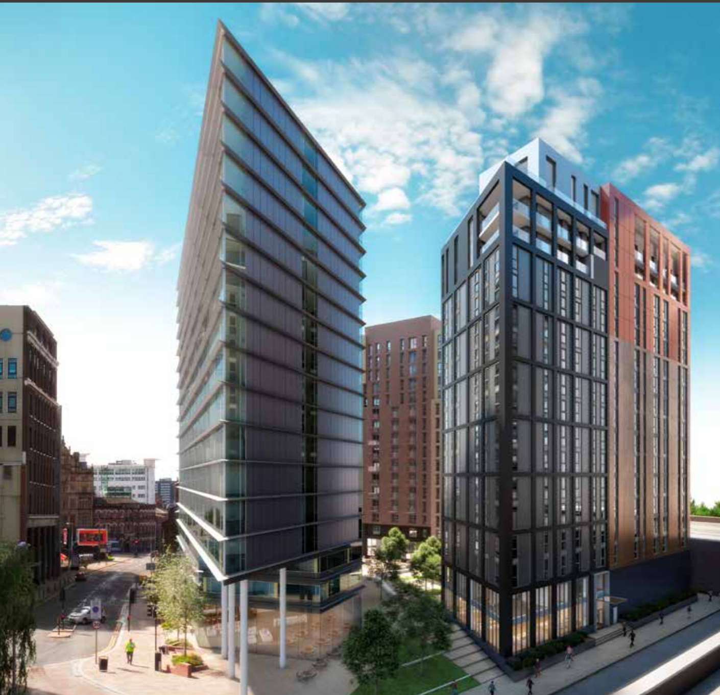
Embankment West, Salford
