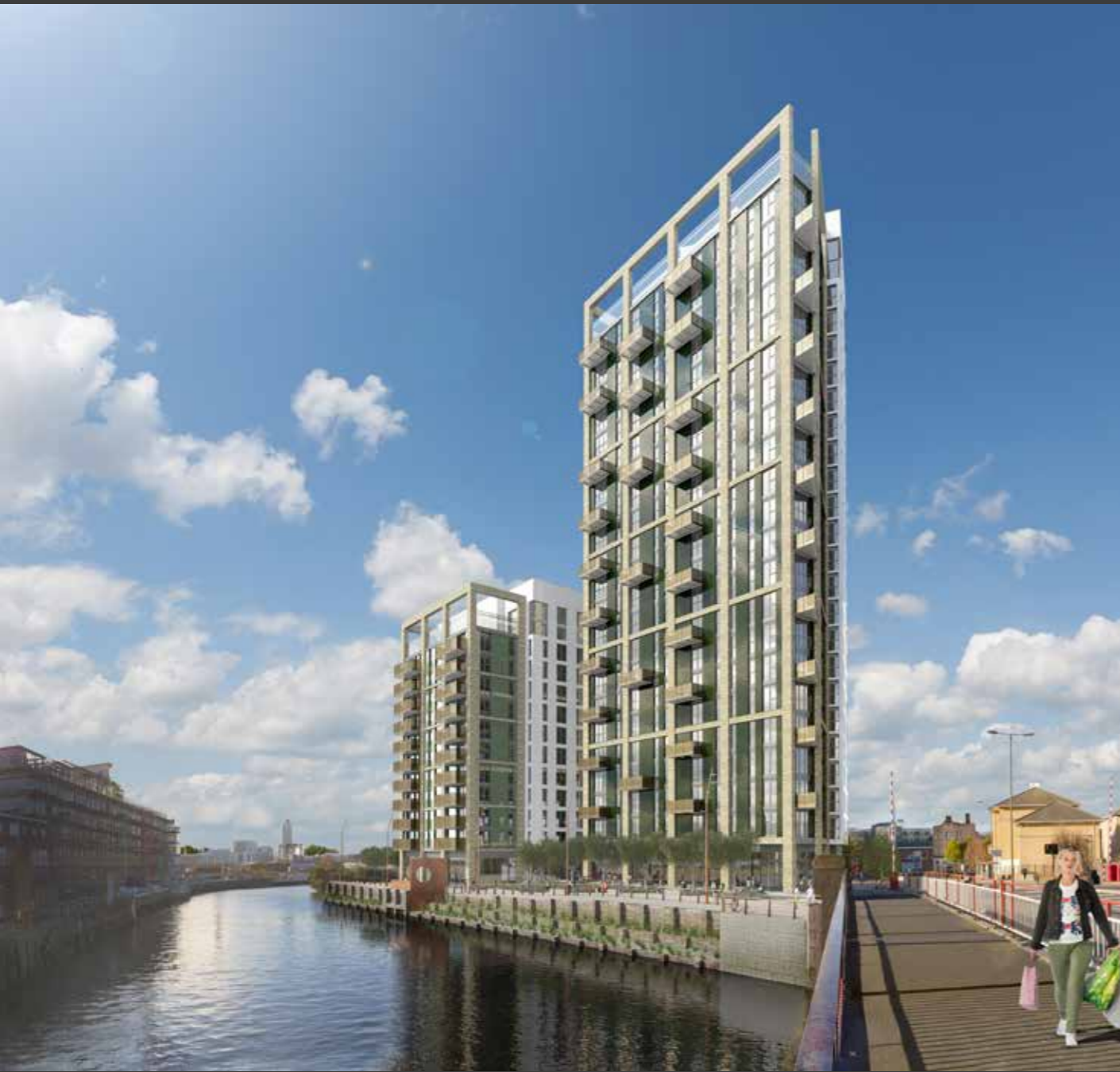
Creekside Wharf, Greenwich
