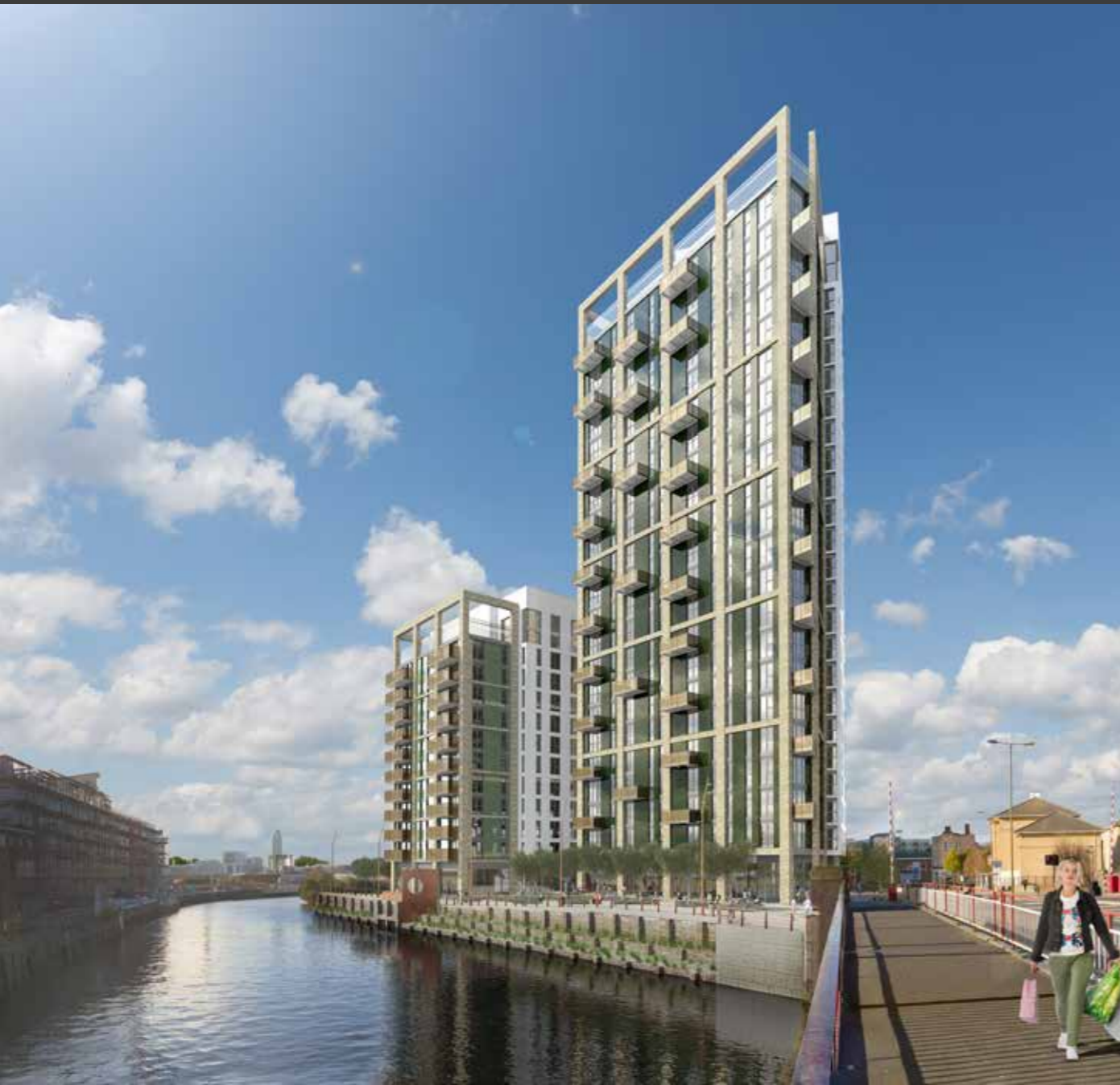
Creekside Wharf, Greenwich
